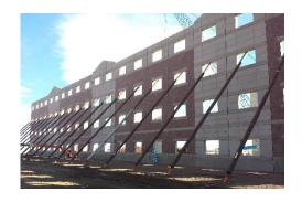
The structure's exterior is clad with prestressed 14-3/4" in. thick insulated wall panels with cast-in conventional clay thin brick accented with acid etched, architectural concrete banding. These panels were combined with fully acid-etched panels to accentuate specific building elements. The versatile precast wall panels provide lateral shear load resistance and support a steel frame floor and roof system.
