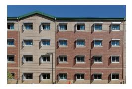
The wall panels are designed to house a significant number of windows to maximize daylight. Because the exterior walls are precast, the windows are anchored within the rough opening cast into each panel. The precast walls contribute to sustainability and high energy performance in the buildings.
