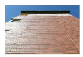
This project features load-bearing precast/prestressed concrete panels, supporting a steel framed floor and roof system, and designed to meet blast loading and antiterrorist-force protection criteria. All panels (207,700 sf) were erected in approximately 15 weeks, dramatically faser than any other exclosure system. The walls contribute to sustainability and high energy performance in the buildings.
